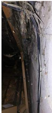
3. Junction between single storey roof and two-storey building
