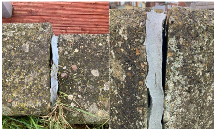
Figure 20: Wall settlement and joint failure in concrete walls.
