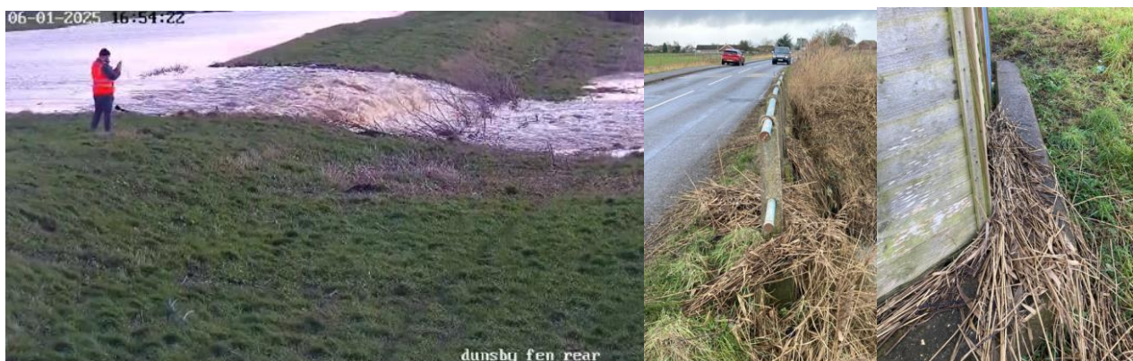
Figure 22 – Evidence of overtopping on South Forty Foot Drain – L to R (and U/S to D/S) Dunsby left bank overtopping, Chain Bridge Road right bank wrack marks on bridge railings, Boston right bank, wrack marks on walls to rear of Wyberton West Road.
