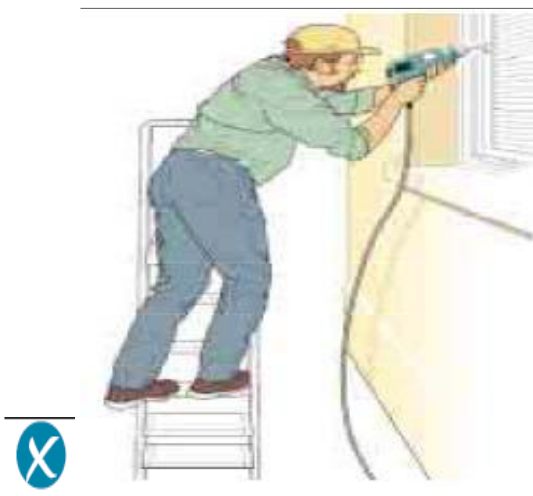
Incorrect – steps side on to work activity
